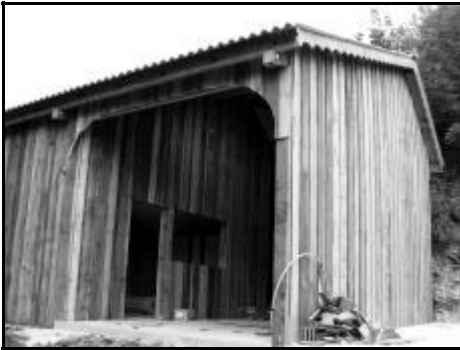
In two weeks we had the shell of what was to become the new hospital with a concrete floor that extended into the area for the release aviary. â
