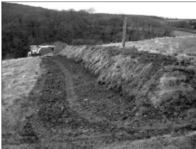
Our contractor faced the bank with scraped-up turf - the disturbed ground should be great for wild flowers
