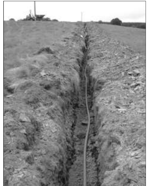
The power cable in the trench Photo: David Ramsden
